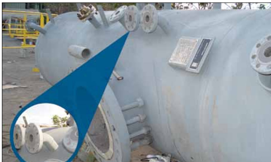
Process vessel shapes can prove difficult to coat and inspect.
