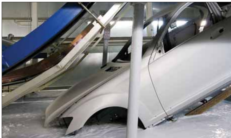
Figure 2: Bottom mounted conveyor EC dip system.
