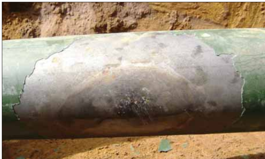
Failure of an external pipe coating system prior to backfilling.
