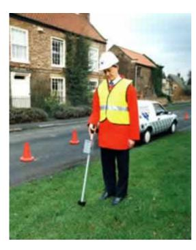
Live cable locators can only find electrical cables that have a current flowing through them to a depth & radius of 5 metres. They will not locate cable through which no power is being drawn.
